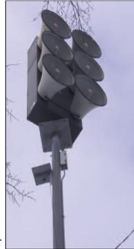
**Fire:** Siren is "on" for 16 seconds, "off" for 8 seconds. Cycle repeats for a 1 ½ minute duration. The "off-on cycle" results in a shrill high-low pitch for 1 ½ minute duration.
